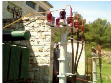
Image 8 Bracket of support insulators, surge arresters and cable terminals on a 35 kV side of the power transformer
