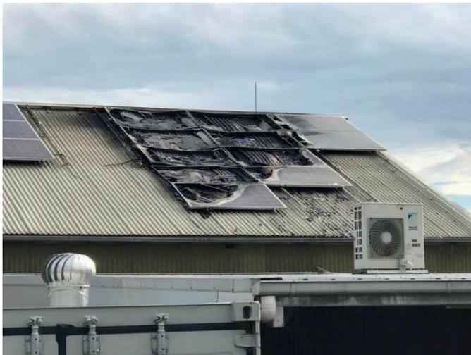
Figure 14. The consequence of fire on photovoltaic system, example, [10]
