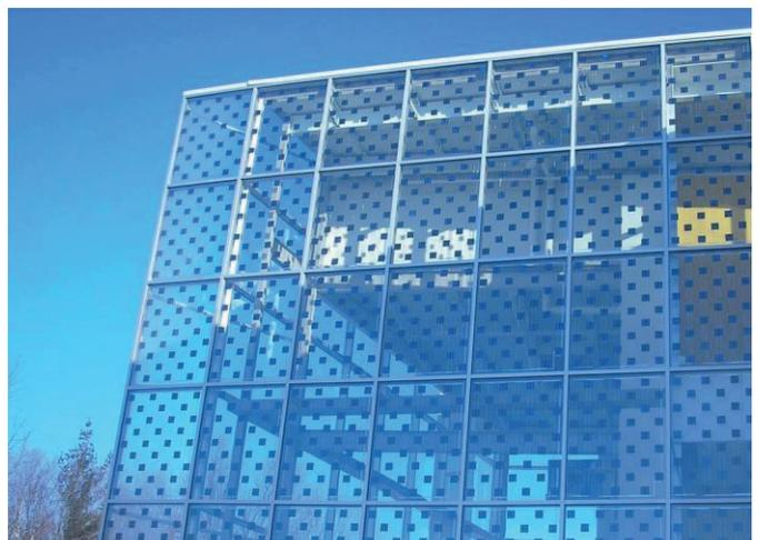
Figure 4. Photovoltaic elements integrated into the façade, [5]
