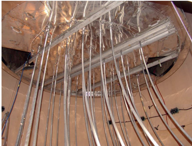
Figure 7: NPP Krško RPV insulation details (1) - inspection openings
