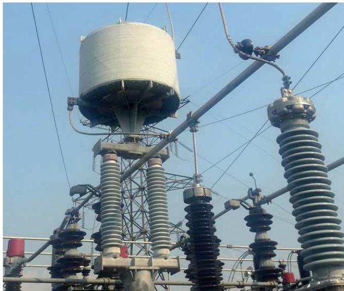
Figure 12. (a) Isometric view of the rigid tubular buswork system, (b) Tubular rigid conductor installed between two disconnectors and going in-between two post insulators for line trap installation
