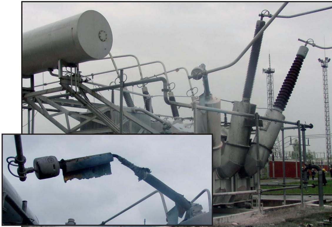
Figure 9: Bushing terminal failure in 2003 and traces of fire on the 300 MVA, 400 kV autotransformer; The right-hand bushing in the figure was replaced after an incipient failure in 1994. Detail shows the bushing debris and the tubular connection dilatation compensator
