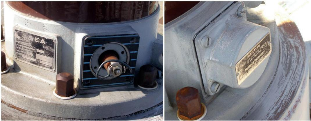
Figure 17 – Measuring tap on ASEA bushing from 1965.
