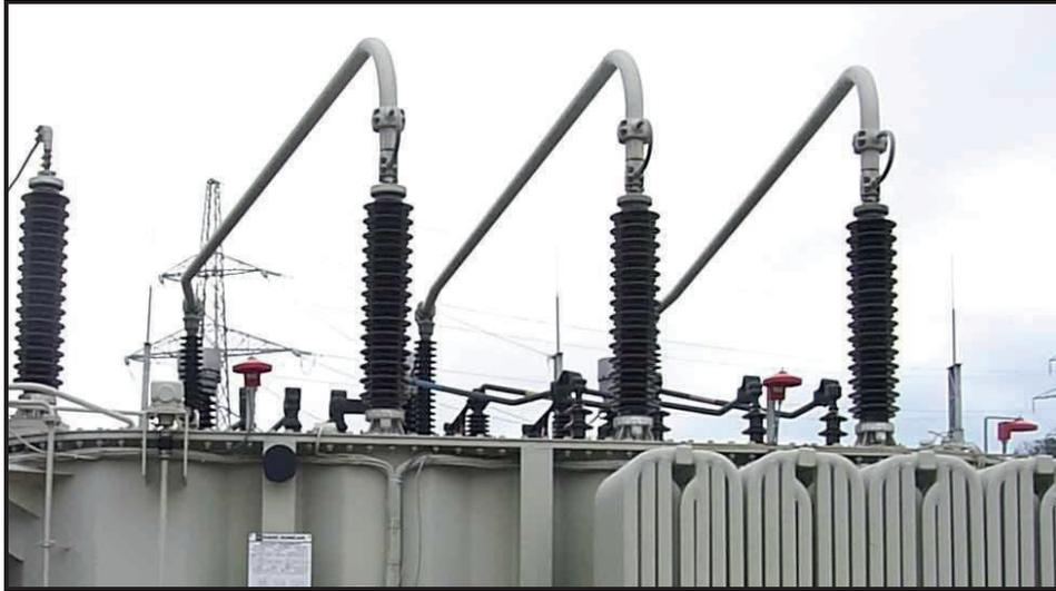
Figure 5: Tubular connections between the switchyard and 123 kV bushings
