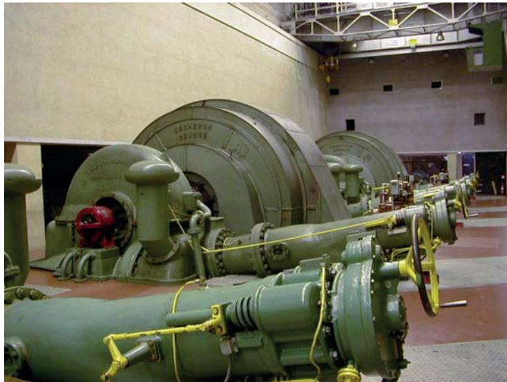
Figure 1 - Hydro-generators (35 MVA) with Pelton turbines
