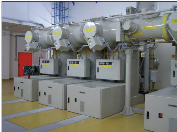
Fig. 2 View on one of the GIS 110 kV substation Dobri in which EMC conditions have been investigated
