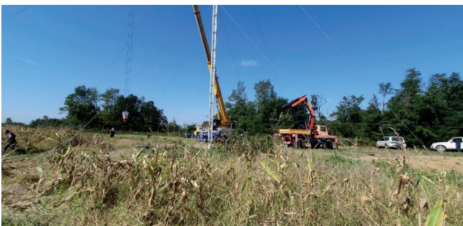
Fig.14. Modular tower installation
