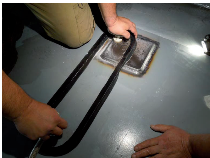
Fig. 6 Vacuum box inspection of welded patch
