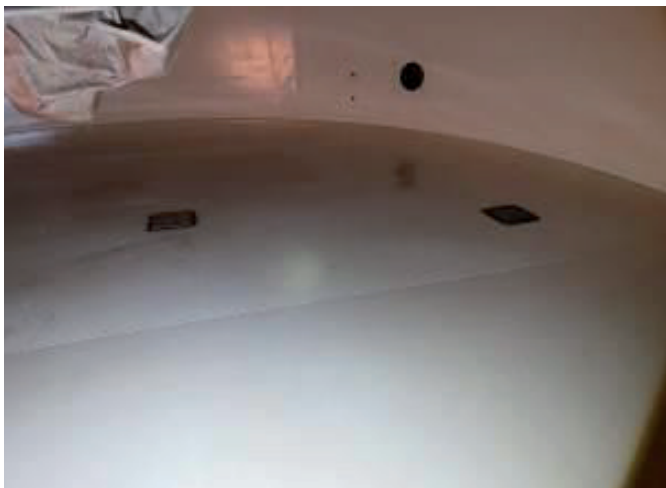
Fig. 14. Steel plates inside CY tank
