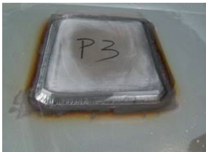
Fig. 12. Steel plate inside CY tank
