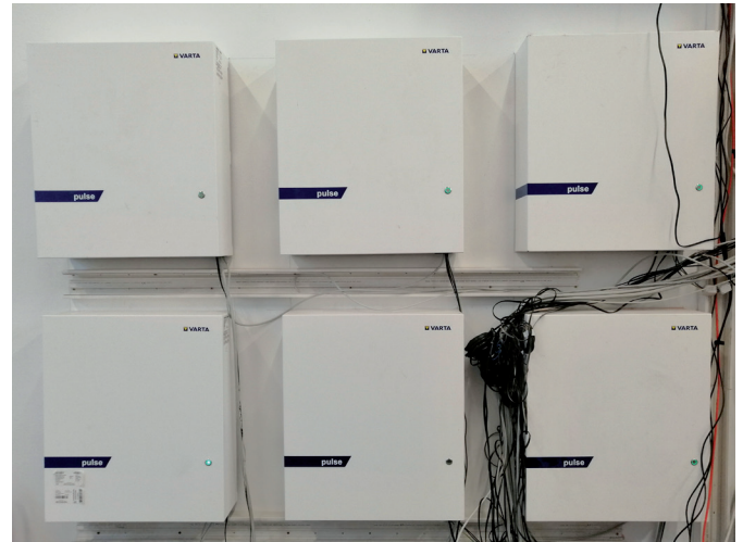
Fig. 2. VARTA Pulse 6 battery units in SGLab
