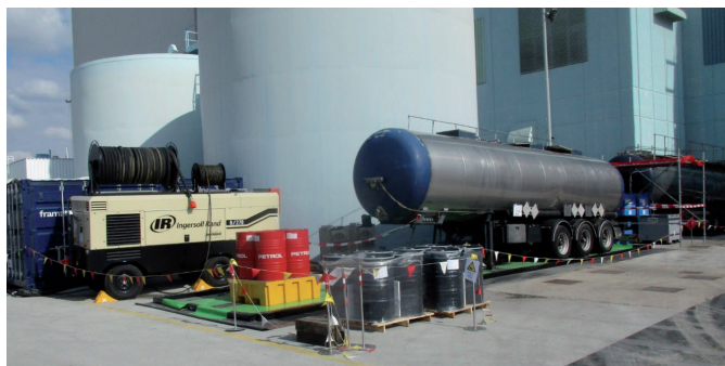
Fig. 2: Equipment setup outside Reactor Building
