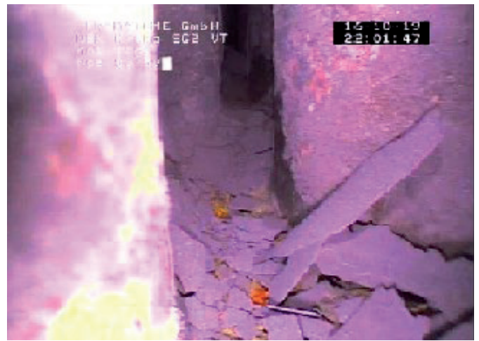
Fig. 11: Fallen scales of magnetite after SG drying phase
