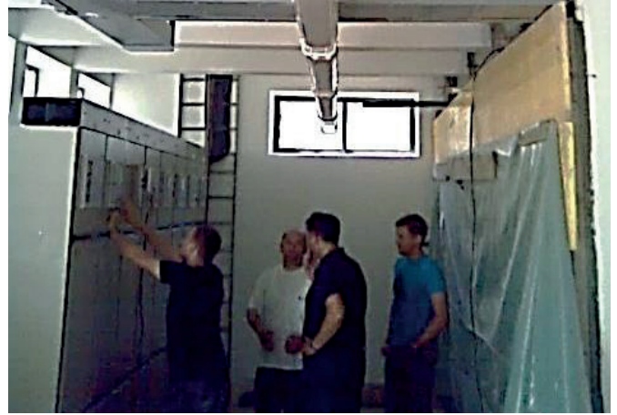
Image 7 Works on the new 10(20) kV plant
