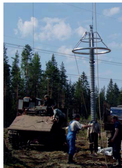
Figure 4. Installation of LSA
