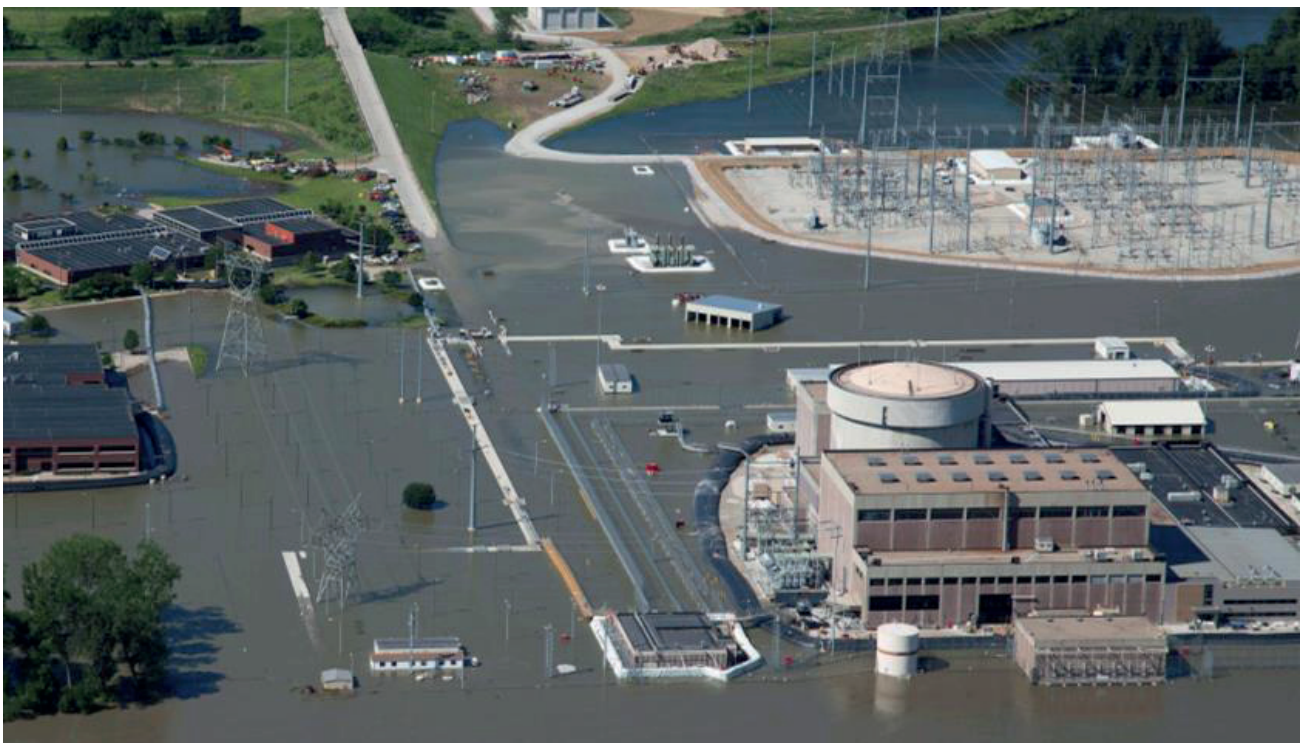
Figure 2 Fort Calhoun plant on 16.06.2011 during the Missouri River Floods; vital buildings were protected using water-filled perimeter "flood berms" (Source: OPPD Public pres., 04.04.2012)
